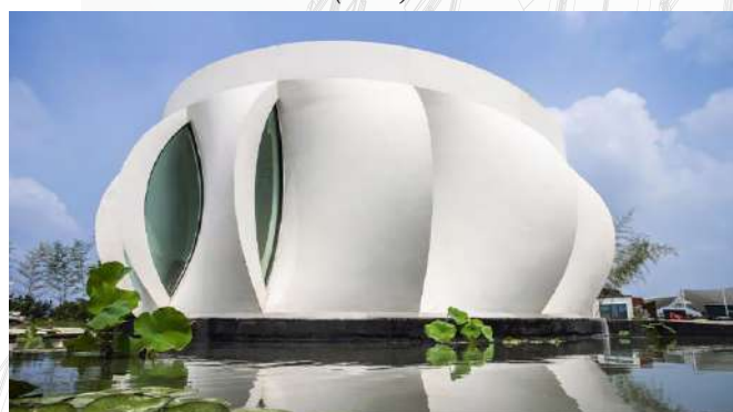
60-square-meter house in Dezhou, China (2018)
